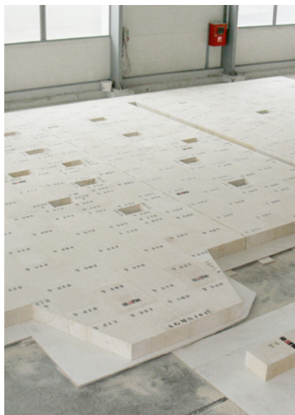
Melting tank fireclay bottom
