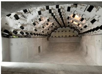
Aluminum smelting furnace during assembly
