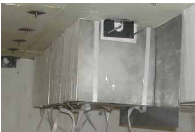
Ceiling mounting of Altra® modules
