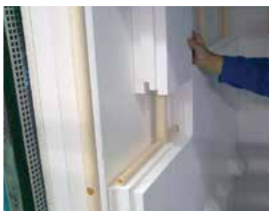
Tongue-and-groove with support system
