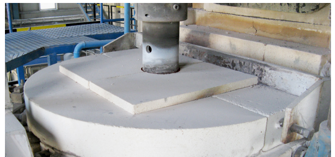
Spout area (burner and cover blocks)
