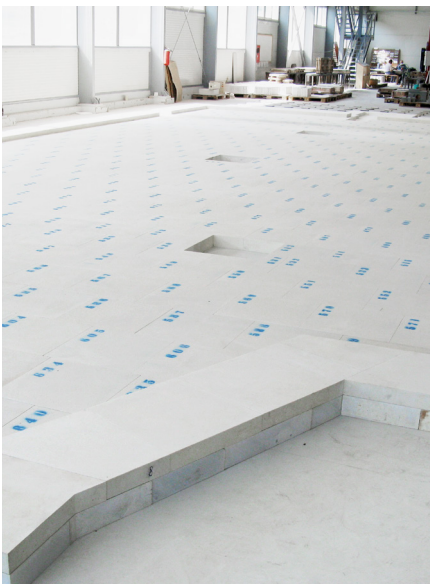
Mullite bottom layer, Oxy-fuel glass melting furnace
