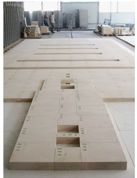
Melting tank bottom with big size light-weight insulation blocks
